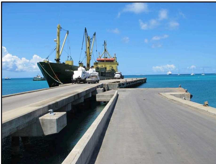
Fig 2 - New Purpose Built RO-RO Jetty
