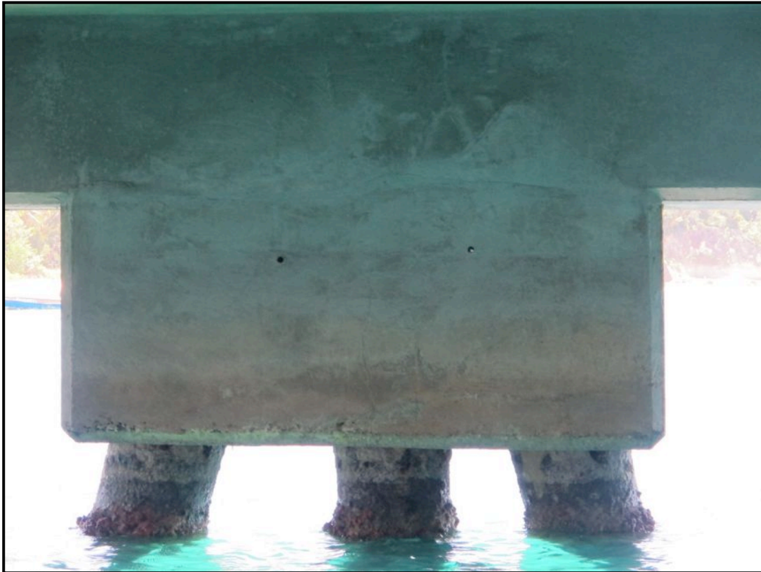
Figure F9 – Underside Repair Extension to Pile Cap
