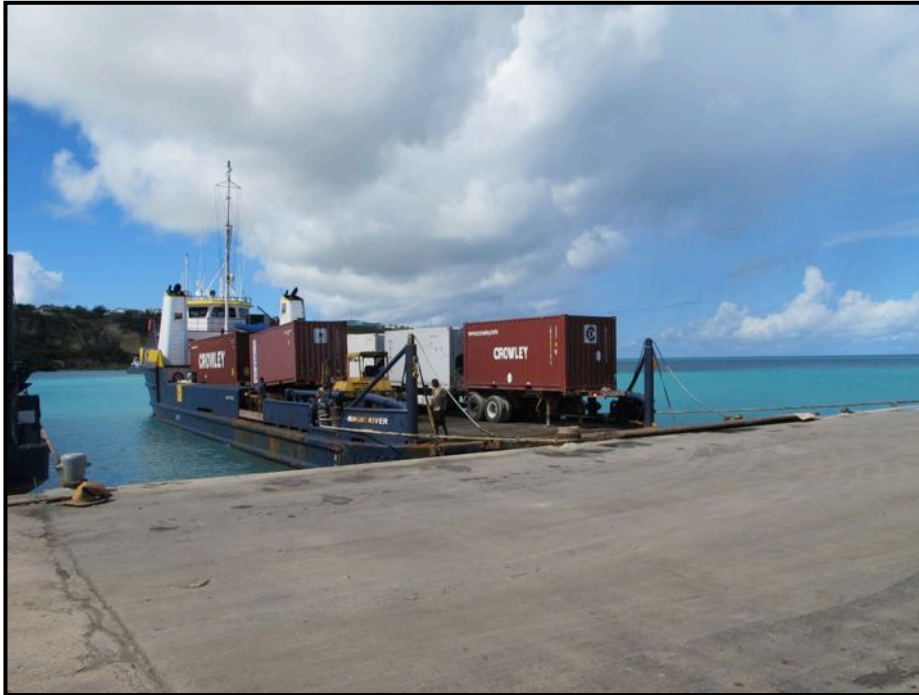
Fig 3 - RO-RO Ship Berthed 'Side-On' to the Jetty
