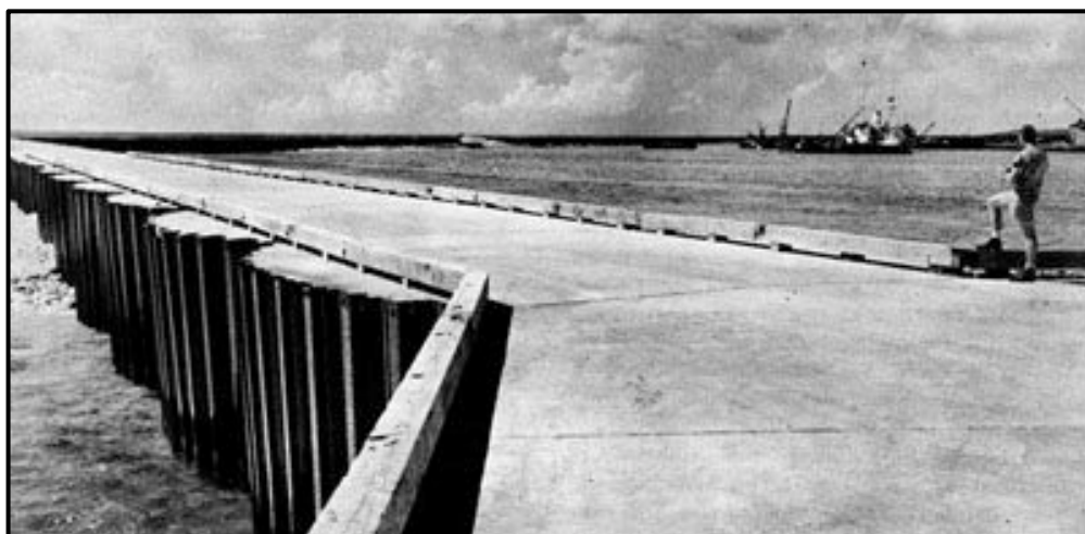
Fig 4 – Example of a Mass Structure Jetty.
