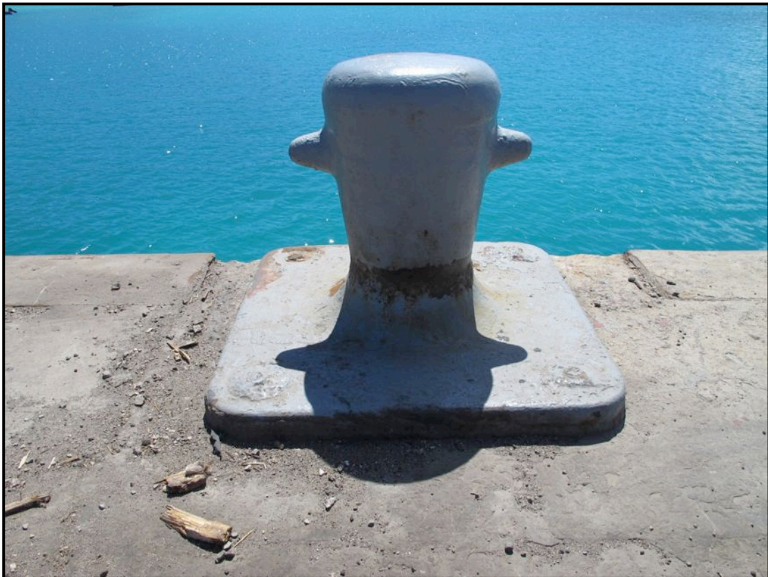
Figure F16 – Mooring Bollard Type 2
